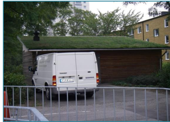
Figure 10 Garage, Augestenberg, Sweden. Source: Alison Duffy
