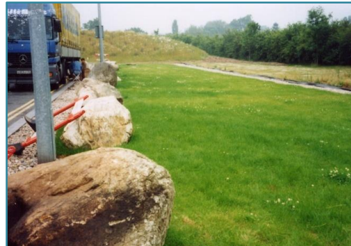
Figure 13 Vehicle lorry park, England. Sheet flow from the car park passes across the filter strip to the filter trench. Source: Fiona Napier
