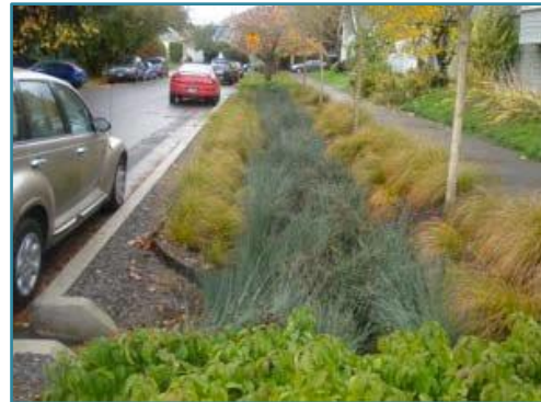
Figure 7 Roadside bioretention in Seattle, USA. Source: Brian D'Arcy
