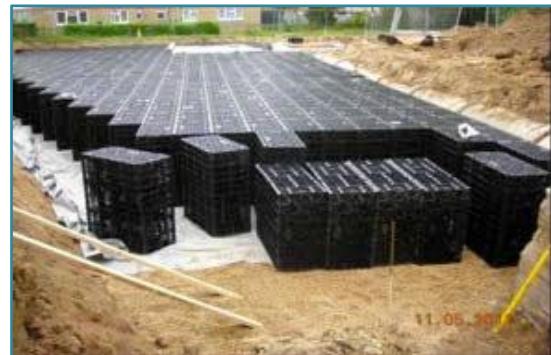
Figure 14 Geocellular units under construction. Source: Chris Digman
