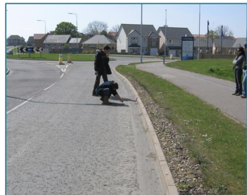
Figure 6 Roadside filter drain, Scotland. Note kerb inlets. Source: Alison Duffy
