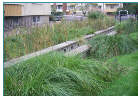
Figure 17 Planted rill in residential area Augustenborg, Sweden. Source: Alison Duffy.
