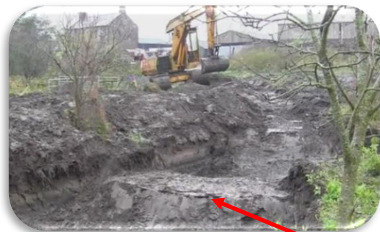
Construction of Pond 1 in 2012 showing berm. Swale in background to the right of the digger
