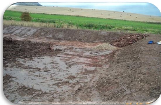
Excavation of the sediment trap bund 2004
