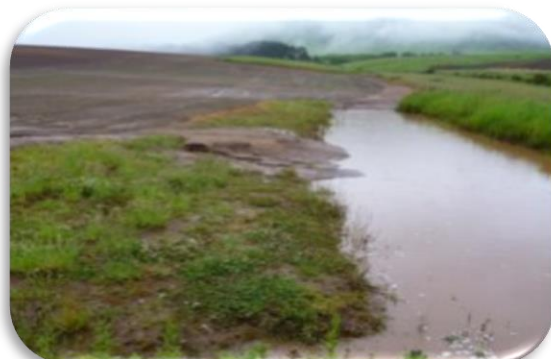
Sediment Trap Bund after heavy rainfall
