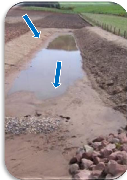
Sediment trap bund in operation
