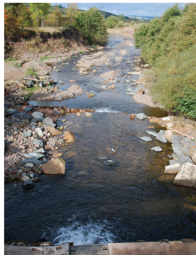
Figure 3.3 The Wooler Water in Northumberland, England. Owing to historical upstream gravel extraction and the use of weirs (shown), the lower part of the river has been starved of coarse sediment leading to unnaturally severe channel erosion (© Natural England).
