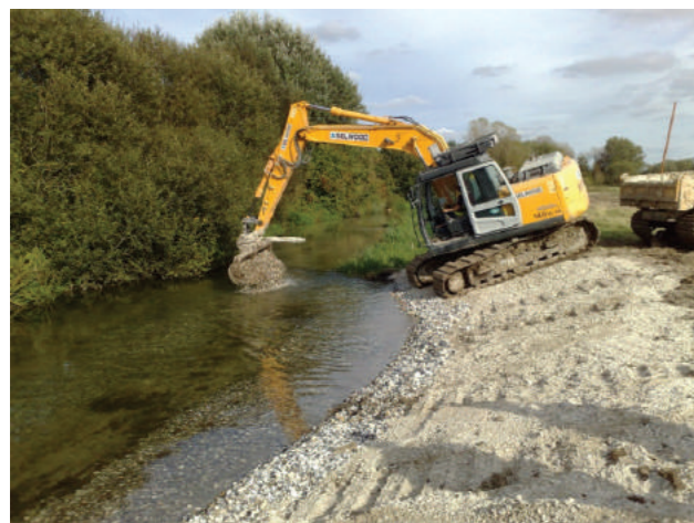
Figure 5.6 (Left) Adding locally sourced gravel to the River Wylve in Wiltshire. This can restore river-bed levels, floodplain connectivity and flow velocities for spawning fish, macroinvertebrates and plant communities (© Hampshire Aquatic Services). (Right) The Ben Gill and River Ehen in Cumbria. The Ben Gill was reconnected to the River Ehen in 2014 to restore natural flows and sediment supply (© Baptiste Mareau, Northern Rivers Institute).
