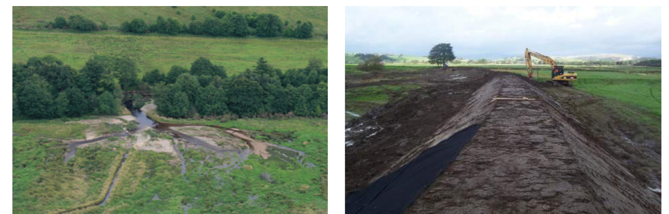
Figure 5.4 (Left) Burn of Mosset in Moray. Breaching a flood embankment has reconnected the channel to its floodplain and led to the development of complex habitat (© Scotavia Images). (Right) Setting back a flood embankment to allow the River Ribble, in Lancashire more space to spill and interact with its floodplain (© Environment Agency).
