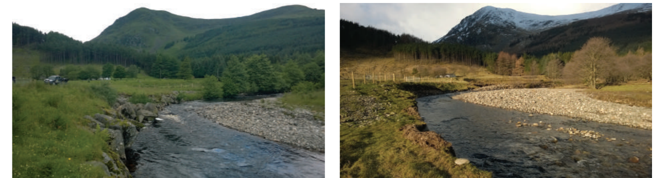
Figure 5.3 (Left) Before and (Right) five months after removal of a section of a boulder protected bank to restore natural channel movement and river-bank habitat on the White Water, Angus (© Kenny MacDougall, EnviroCentre).
