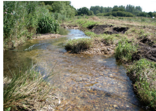
The River Tat, a tributary of the River Wensum, (Left) before and (Right) after bank re-profiling and gravel placement in 2010 to restore channel sinuosity and varied river-bed levels (© Adam Thurtle, Environment Agency).
