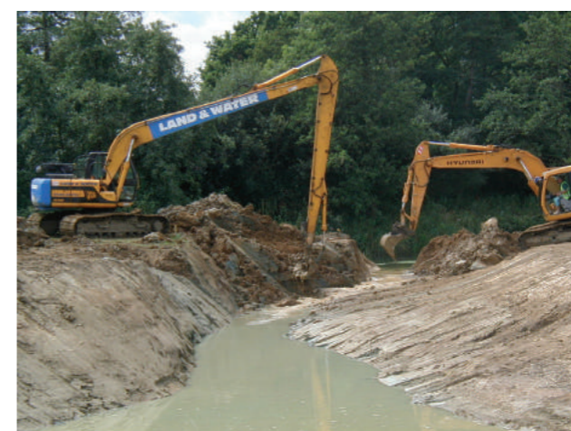
Figure 5.12 Excavation to reveal and reconnect the old meander loop at Shopham on the River Rother, West Sussex in 2004 (Left) and (Right) the newly reconnected meander (© Damon Block, Environment Agency).
