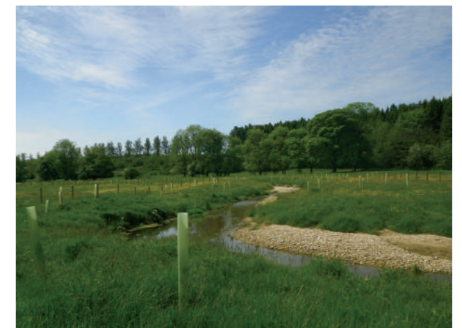
Figure 5.11 (Left) Aerial view of the River Lyvennet and Howe Beck, Cumbria in Autumn 2014 after re-meandering and diversion from the previously channelised rivers resulting in nearly 2 km of new river habitat (© Oliver Southgate, Environment Agency). (Right) The Howe Beck nine months after excavation and diversion along the course of an old channel (© Daniel Brazier, Eden Rivers Trust).
