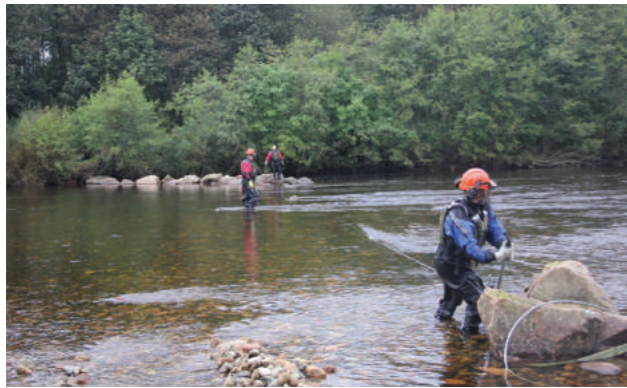
Figure 5.8 Removal of a 'croy' structure (deflector) by using hand winches on the River Dee, Aberdeenshire to restore the continuity of water flow, sediment movement and river-bed habitat (© River Dee Trust).
