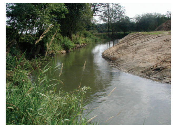
Figure 5.12 Excavation to reveal and reconnect the old meander loop at Shopham on the River Rother, West Sussex in 2004 (Left) and (Right) the newly reconnected meander (© Damon Block, Environment Agency).
