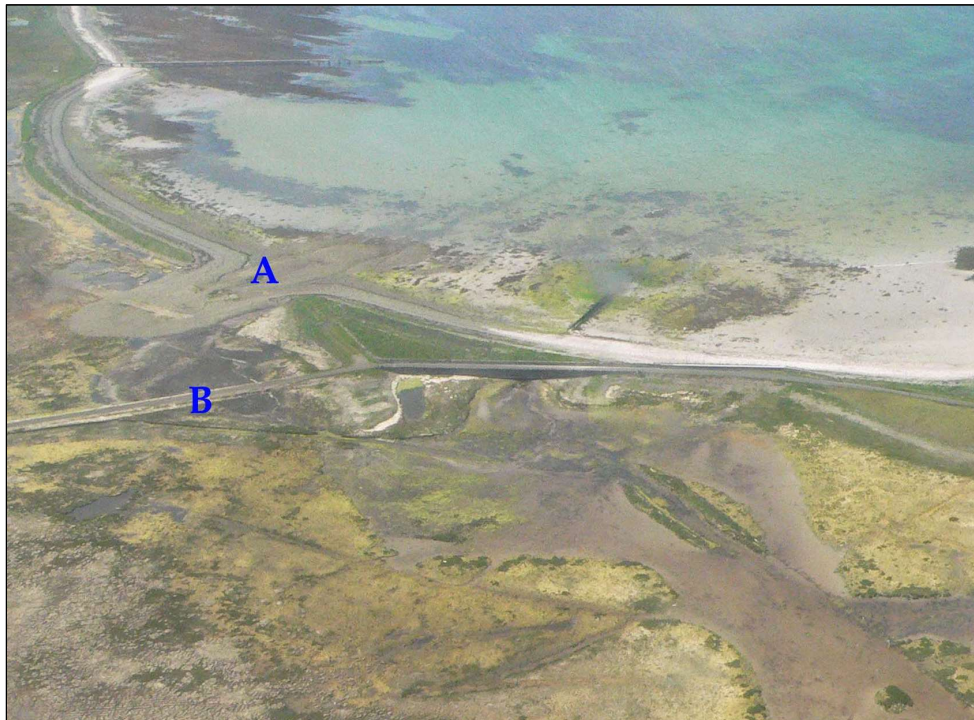
Figure 4.1: Aerial image of breaching, overwash (A) resulting in flooding of road (B) enhanced by low-lying and landward sloping interior (negative gradient). SW of Cleat, Little Sea, Sanday, Orkney.
