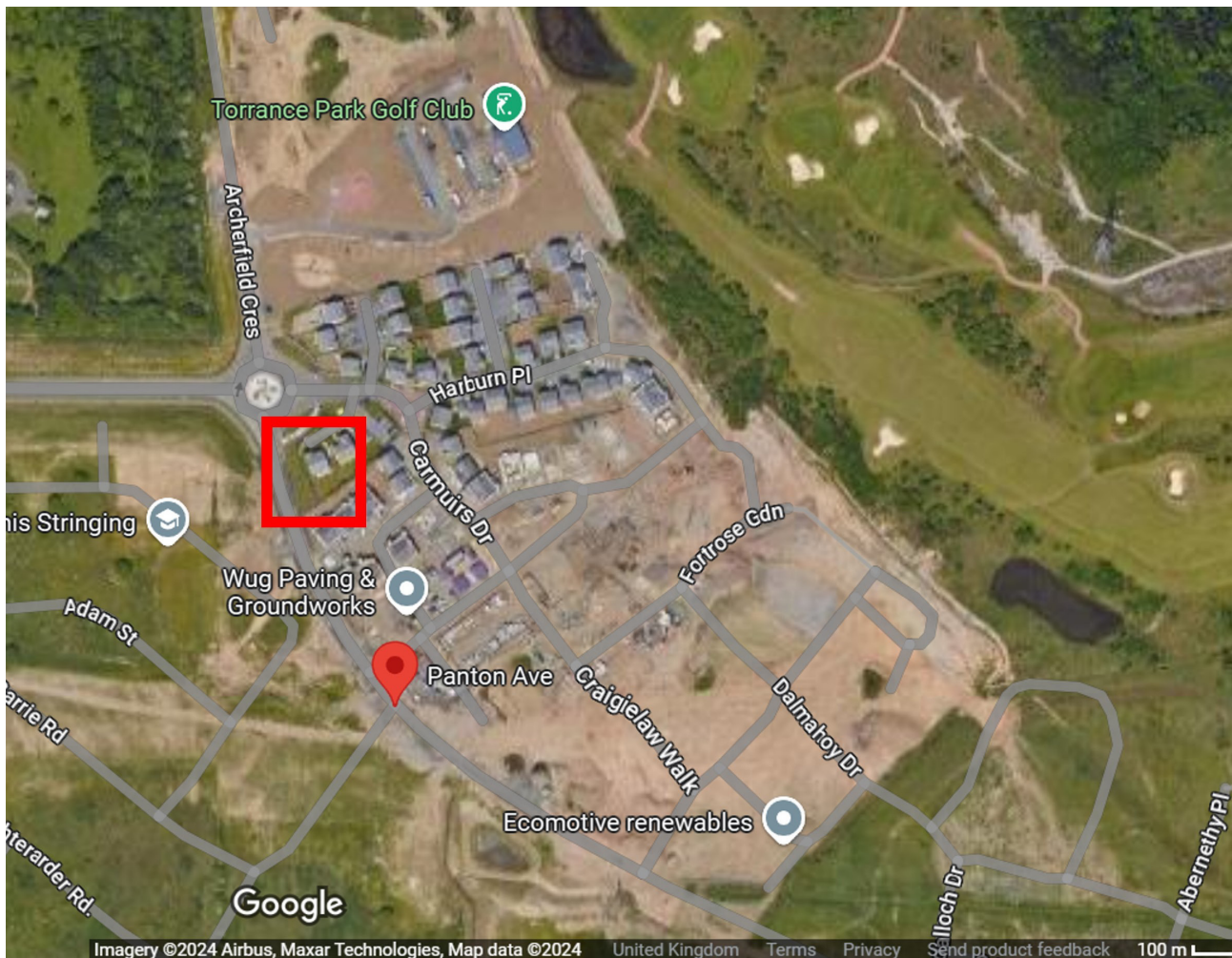
Figure B2.1. The Taylor Wimpey showhome location (highlighted in red) at the Holytown site. Image source: Google Maps.
