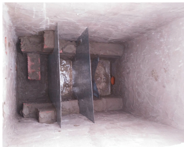
Figure B2.4. In-ground attenuation device design (left) gully guard sack (right). Image source: James Travers.
