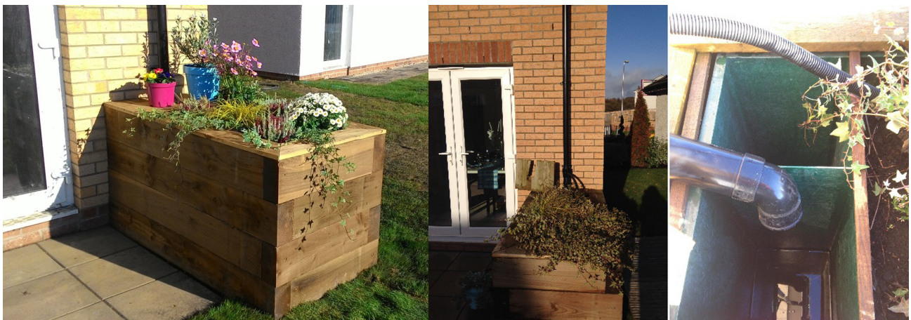
Figure B2.2. Boxed raingarden at the show home (left) and the disconnection of the downpipe into the multi-cell box (right). Image source: James Travers.
