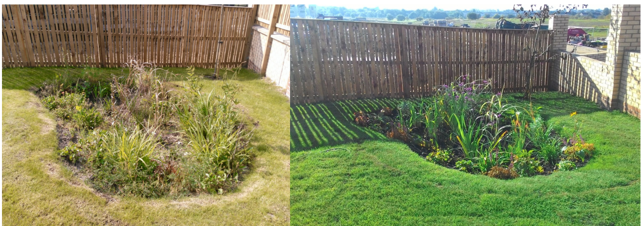
Figure B2.3. In-ground raingarden at the show home. Image source: James Travers.
