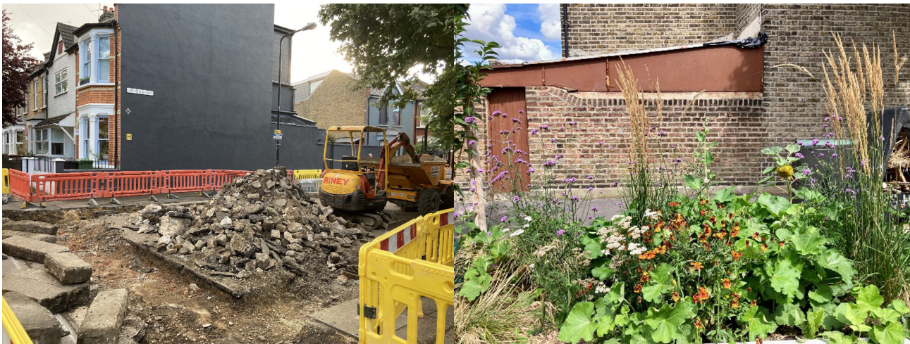
Figure B4.3. Excavation for raingardens (left) and variety of plant species for colour and texture incorporated in the raingardens (right). Image source: Tom Fewins.
