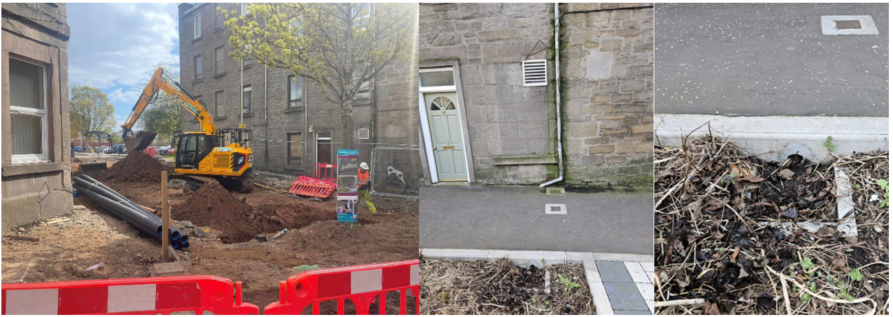
Figure B1.11. Construction of the raingardens (left). Downpipe disconnection into the raingarden (right). Image source: Stobswell Forum SCIO (left) and Abertay University (right).
