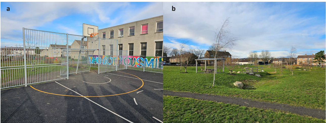
Figure B3.4. Community Park surface water management solutions: (a) permeable paving surface to basketball court; and (b) swales. Image source: Scottish Water.
