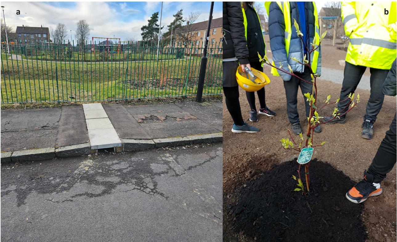
Figure B3.3. (a) Drainage conduit from public carriageway into Community Park. (b). Local primary schools planting trees in the Community Park. Image source: Scottish Water, courtesy of Claypotts Primary School, Dundee.
