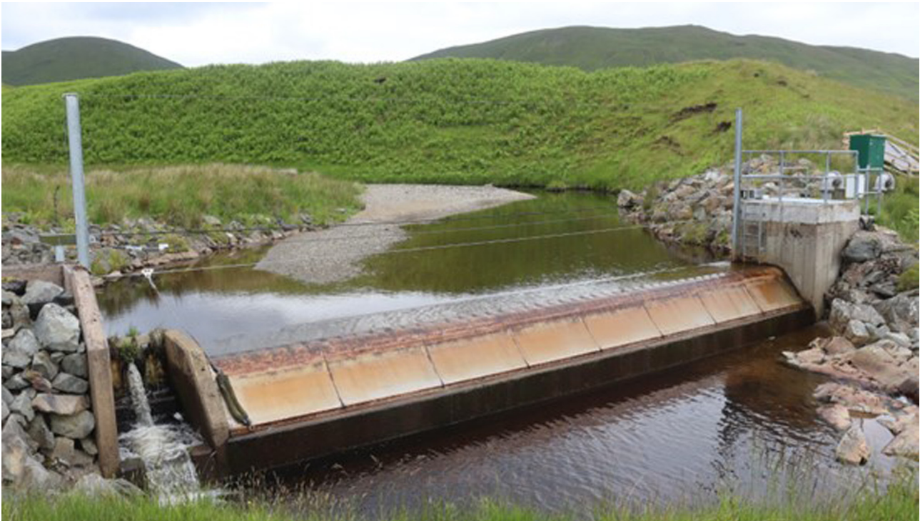
Figure 1 – Hydro impoundment (Photograph courtesy of Richard Williams).
