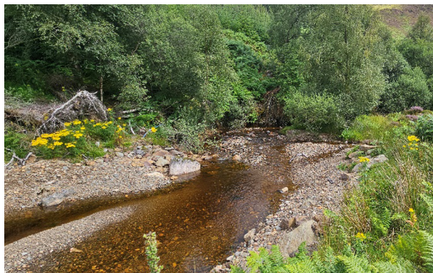
Photo 3D Sediment accumulation behind impoundment. Looking upstream. Taken from river left.
