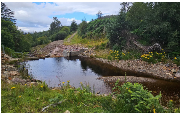
Photo 3C Headpond and sediment accumulation behind impoundment. Looking downstream. Taken from river left.
