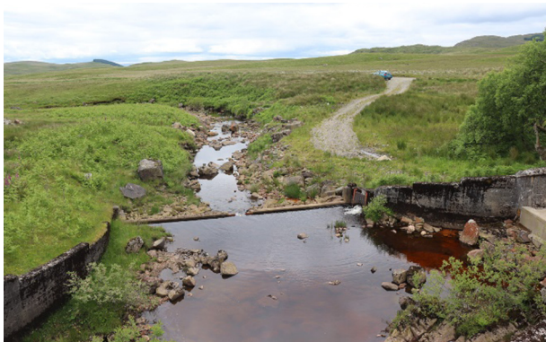
Photo 1E Impoundment. Looking downstream. Taken from impoundment.
