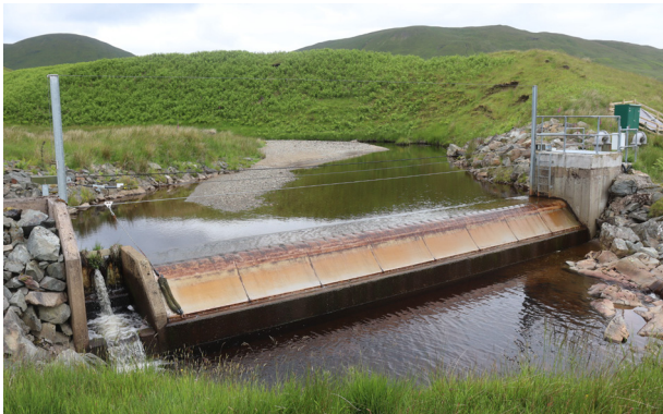
Photo 2A RoR impoundment. Looking upstream. Taken from river right.
