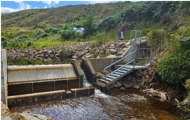
Photo 3A RoR impoundment. Looking upstream. Taken from river right.
