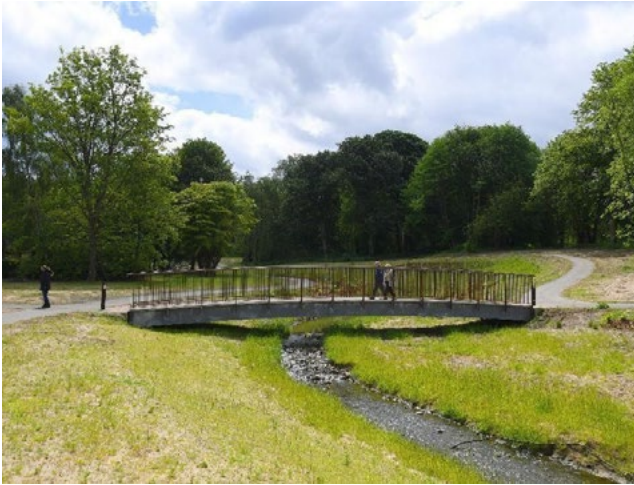
Figure 5 - New footbridge over Tollcross Burn
