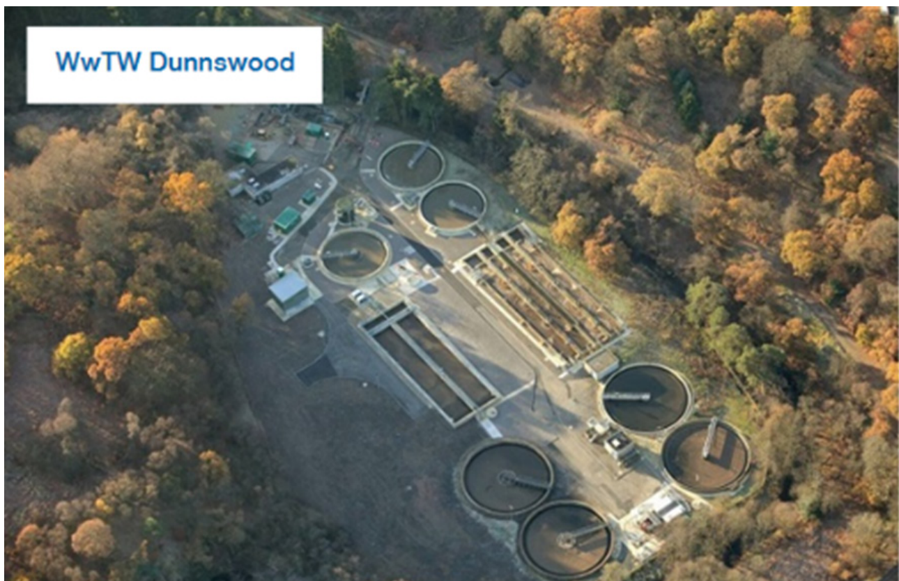
Figure 6. Image of Dunnswood WWTW.
