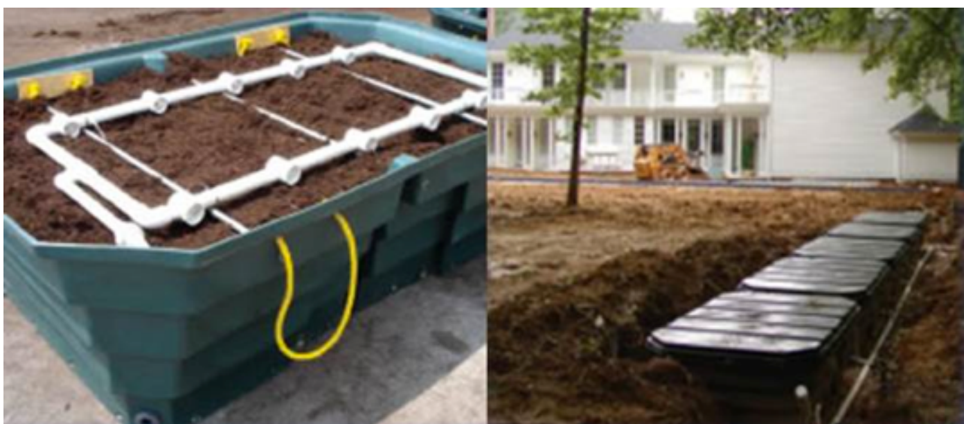
Figure 10 Puraflo peat biofilter system from Bord na Móna (Flemington Precast & Supply, L.L.C. 2014).
